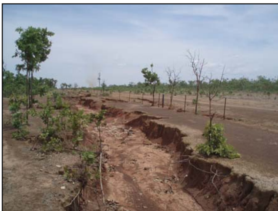
Photo 1: Fenceline erosion within the Darwin Pastoral District.
