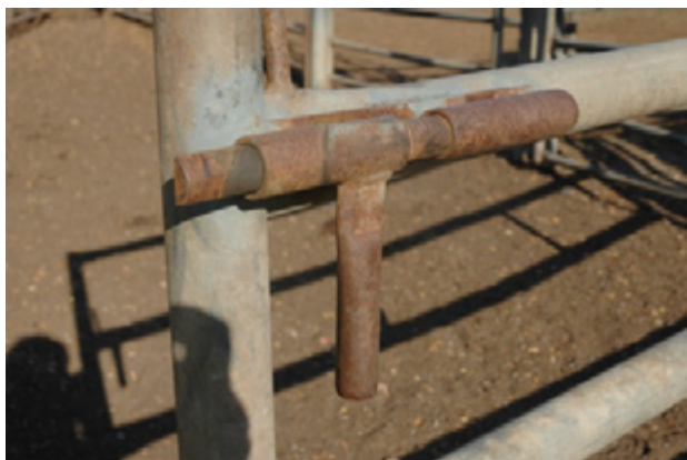
Figure 11.11 Spring-loaded gate handle. The gate will lock instantly and safely when slammed shut, not requiring the operator to be close by.
