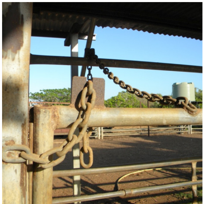
Figure 11.5 Vee race restraining chains. These chains determine the position of the front bottom-hinged panel. To close up the panel for smaller stock, the left hand chain is lengthened and the higher, longer chain at the top is shortened.
