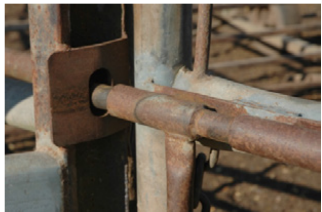
Figure 11.11 Spring-loaded gate handle. The gate will lock instantly and safely when slammed shut, not requiring the operator to be close by.
