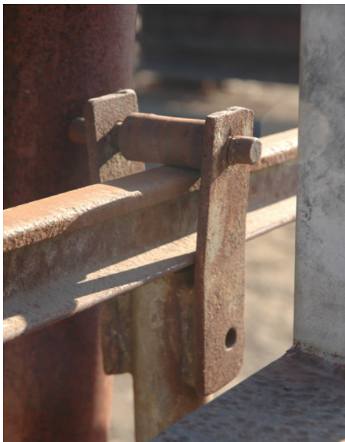
Figure 11.12 Sliding gates can be made quite simply. On the left is the upper slider, two of which are needed. On the right is a swinging gate that does a similar job to a slider for smaller applications such as on this calf cradle.
