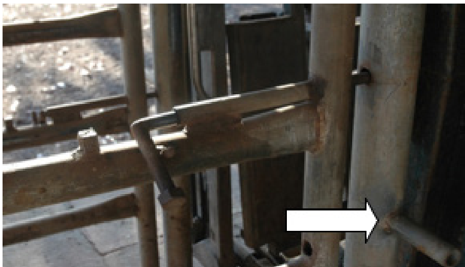
Figure 11.14 A station gate latch made from readily available materials. Arrowed is one of three pipe lugs of heavy-walled 25 mm galvanized pipe, 100 to 150 mm in length fixed about 200 to 250 mm apart in parallel, fillet-welded to the stationary crush framing or roof support post next to the head bail for attaching ropes used for restraining the buffalo's head for horn tipping, blood sampling etc.
