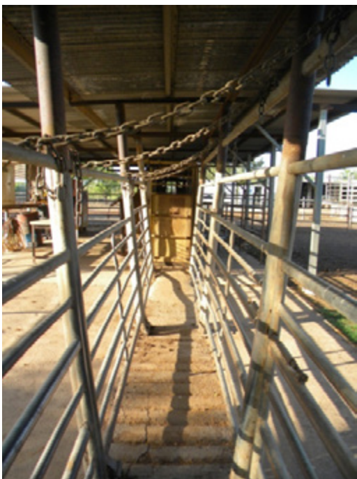
Figure 11.4 Example of a Vee race suitable for adult buffalo bulls and cows. This view shows the panels in their widest position. Vertical posts are fixed in position. The RHS panels are side-hinged to open outwards in the event an animal goes down in the race. The left hand panels are bottom-hinged to come in to position determined by the restraining chains. For example, shortening one while lengthening the other will close up the left hand panel.
