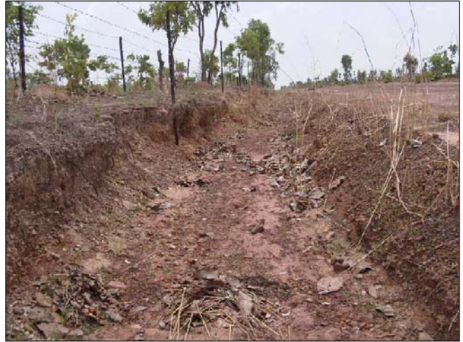
Photo 4: Fenceline and track erosion in the Darwin Pastoral District
