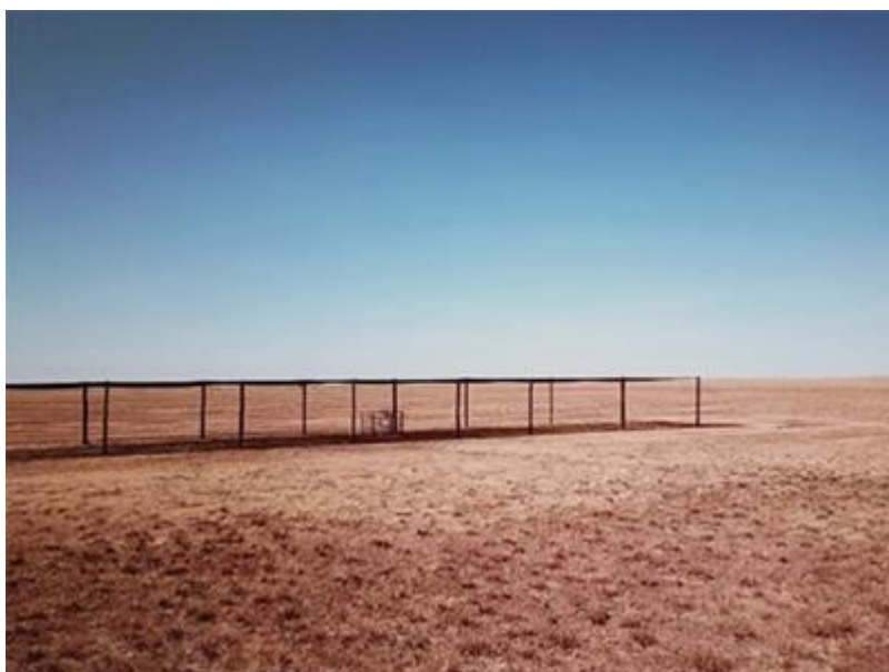
Above: Picture of the shade structure at Avon Downs station.
